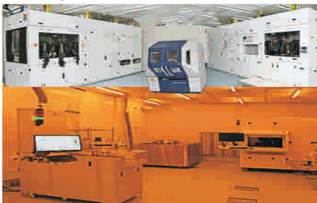
Compound Semiconductor Facility
